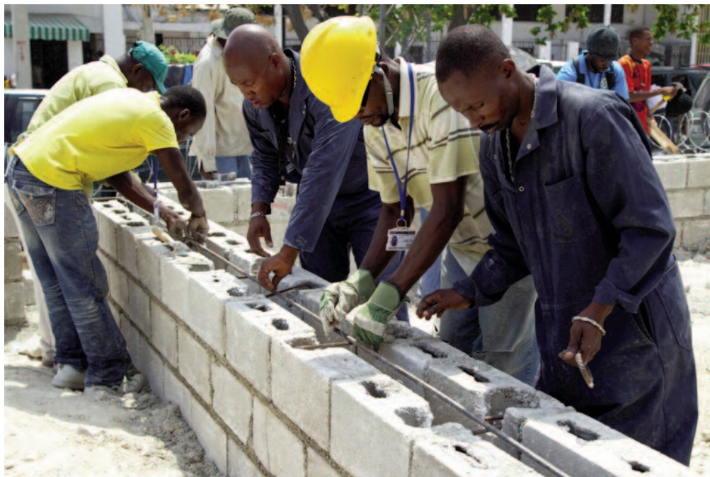
Following the destruction of the Haitian Parliament in the January 2010 earthquake, construction workers build a temporary Haitian Parliament facility with funds from MINUSTAH in March 2011. UN Photo/Logan Abassi.
