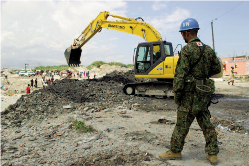
Military engineers from the UN mission in Haiti (MINUSTAH) work to clean debris blocking canals around Port-au-Prince in April 2012, in an attempt to minimize flooding during the upcoming rainy season. UN Photo/Logan Abassi.
